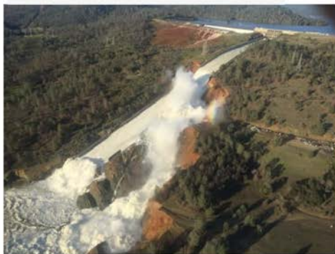
Oroville dam 2017. Photo: City of Oroville
